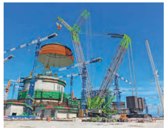
A team from the China Nuclear Industry Mechanical Engineering Co (CNME) hoisted the 487 tonne dome of the No. 1 generator unit at Zhangzhou Nuclear Power Plant in East China's Fujian Province. A 3,200 tonne capacity Zoomlion ZCC3200NP lattice boom crawler crane owned by CNME (10th place) made the lift
